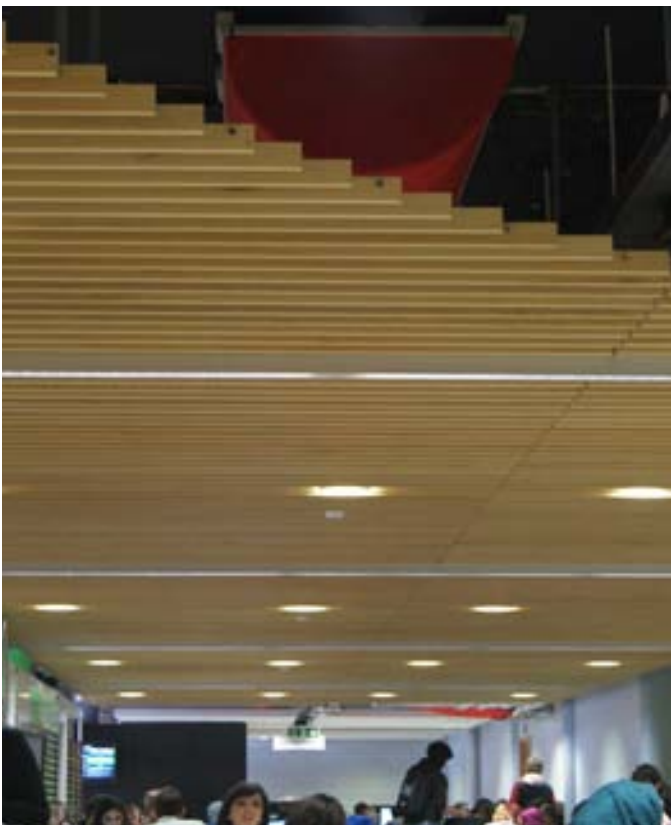
Part of a larger system running the length of a meeting and working area
