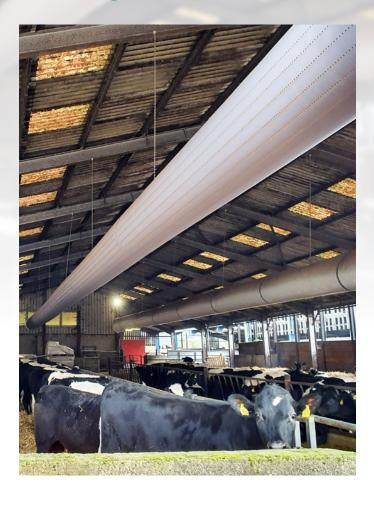
to Prihoda's fabric ducting. For example, the PE tubes could get soiled easily in the dusty conditions commonly present in animal housing. The antibacterial treatment available with fabric ducting was also a desirable feature for this application.
