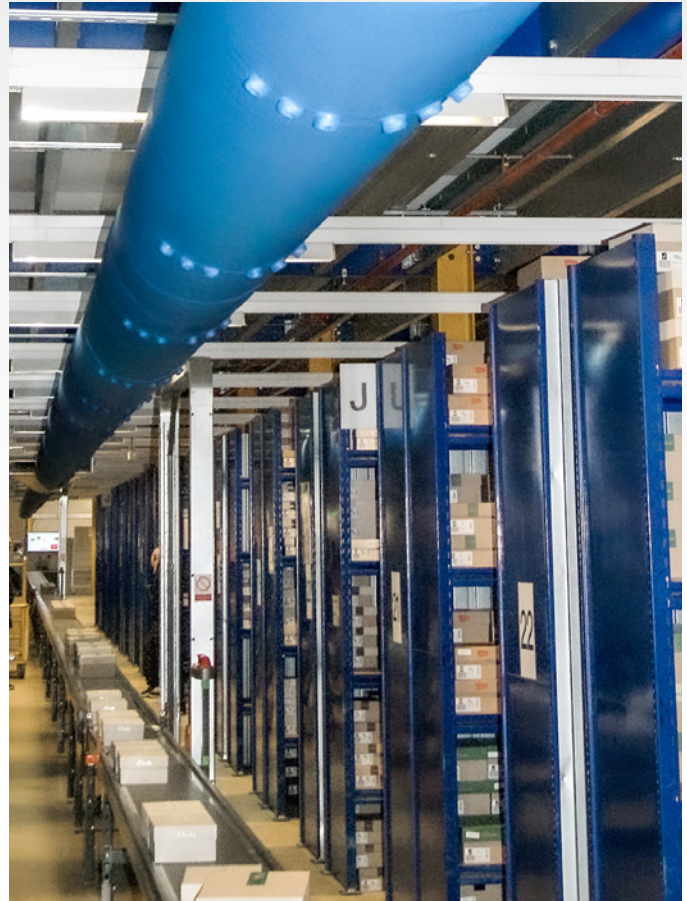
Fabric nozzles direct the air where it is needed.
