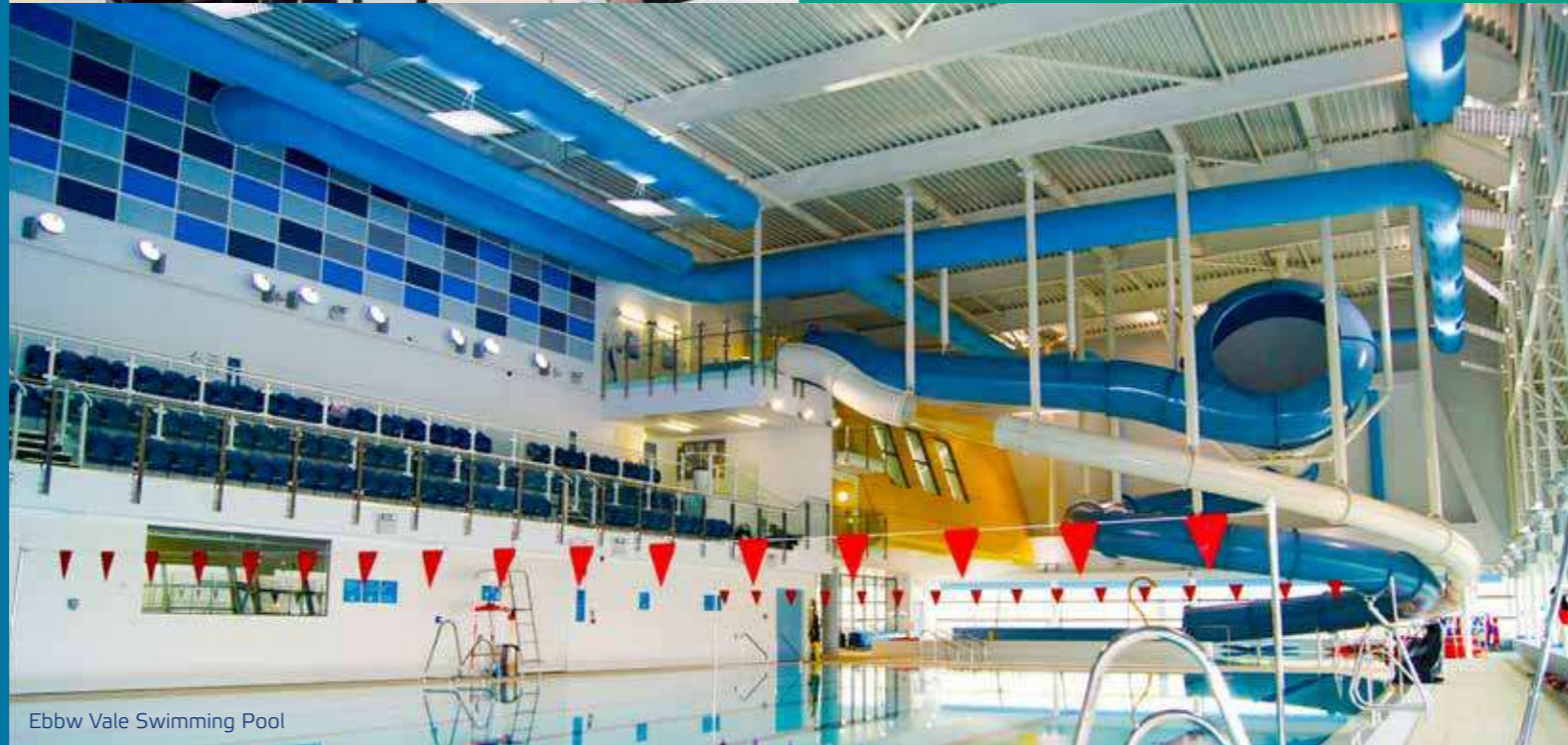
Fabric Ducting with lighting
