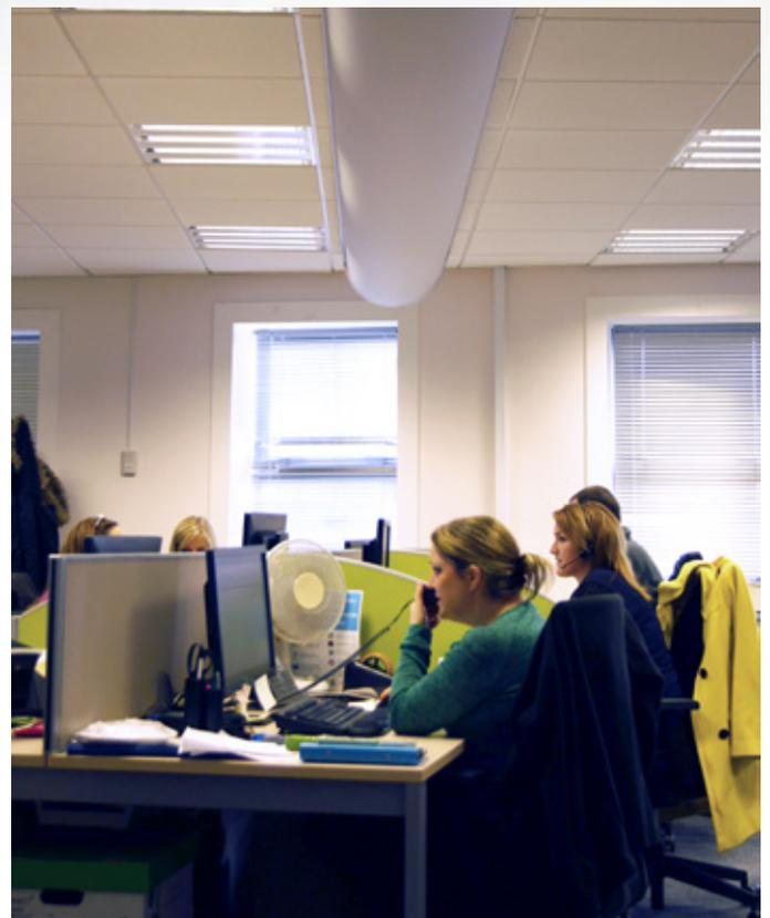
better than imagined and regular complaints about the AC system are now a thing of the past. The open plan floors are comfortable, of an even temperature gradient and velocity free, even with ducts mounted over desks. Our patented micro-perforation diffusers avoid 'dumping' of cold air below the duct, which is unavoidable with permeable material fabric ducts alone (this video link shows a smoke test of this problem <https://vimeo.com/100693994>).
